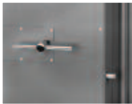
Inside escape mechanism
